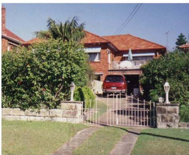
Lewis Street (Before)
